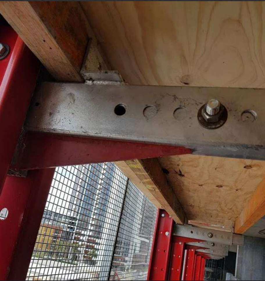
WORKING DECK FROM UNDERSIDE
